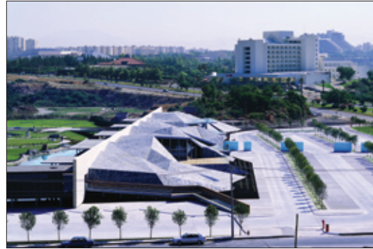
Minicity designed by EAA-Emre Arolat Architects, Antalya, 2004; photo by Cemal Emden
